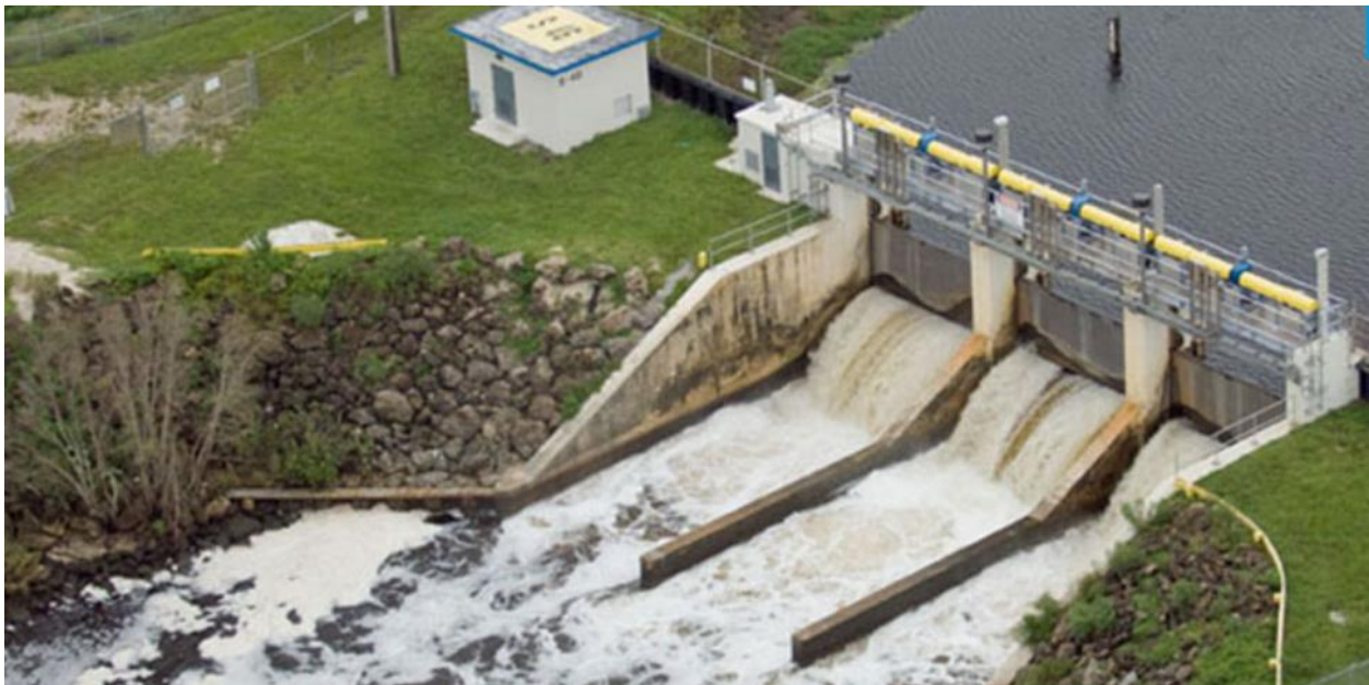
Figure 1. A spillway in the South Florida Water Management District's system of more than 1000 pump stations, weirs, locks, culverts, canals, and levees.
